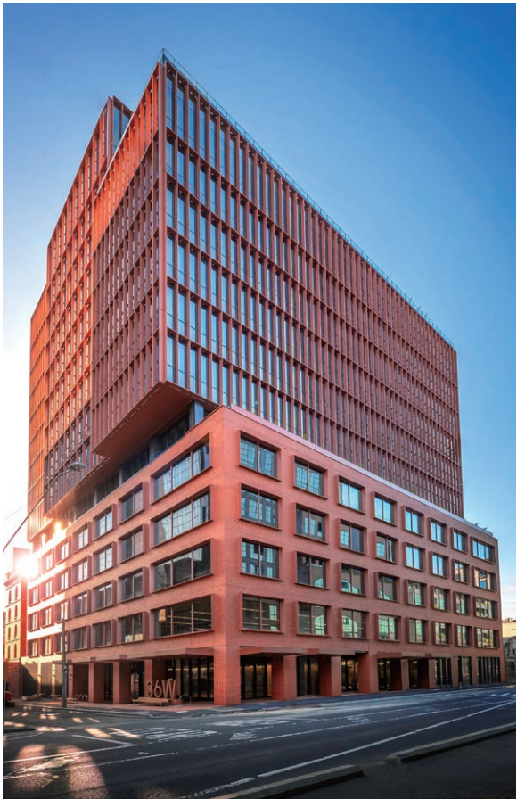
Hybrid structure of reinforced concrete (RC) structure from the 1st to 6th floors, and timber structure from the 7th to 15th floors Tallest completed timber office building in Australia
