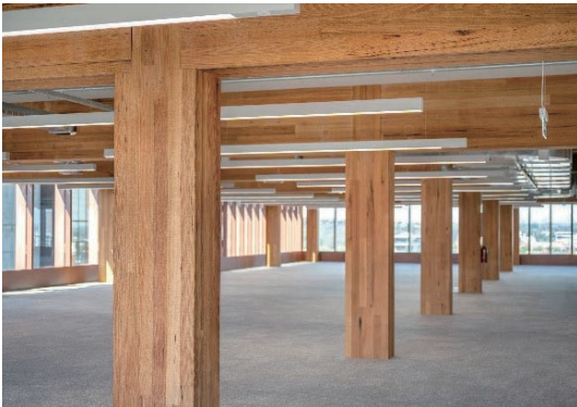
Posts and beams are made from engineered wood produced locally in Victoria Cross-laminated timber (CLT) made from Australian radiata pine is used for the floor slabs
