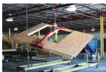
Image of wall panel
