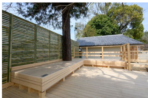
Newly constructed viewing deck; benches are made with Japanese cypress from Sumitomo Forestry-owned forests
